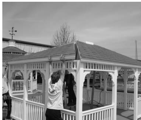
Step 25: Install remaining roof sections placing roof sections with matching numbers.
