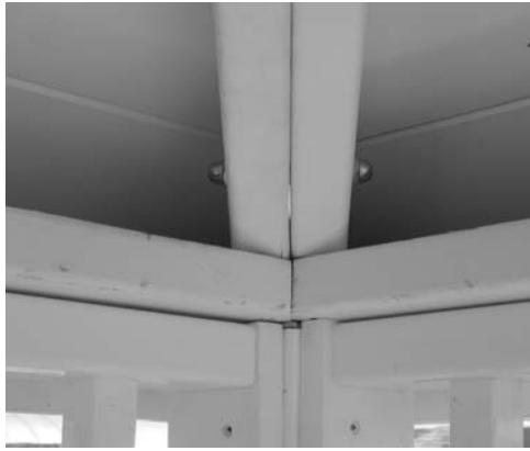
Step 29: Align roof sections and bolt tightly using ratchet set.
