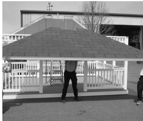
Step 23: Install opposite large roof section repeating previous steps.
