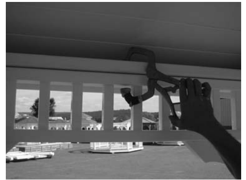
Step 29: Align roof sections and bolt tightly using ratchet set.
