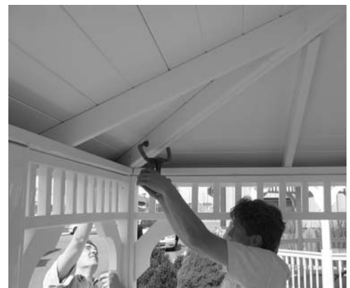
Step 27: Fasten with clamp to temporarily hold roof section in place.
