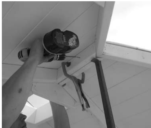
Step 24: Clamp and fasten top ridge beam aligning corners precisely.
