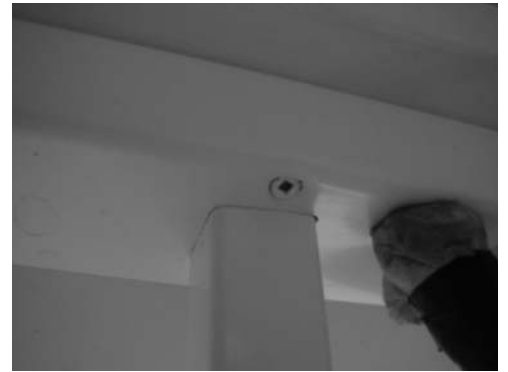
Tip: Do not drive screw too far into vinyl.
