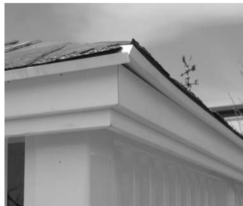
Step 26: Align outside corners precisely.
