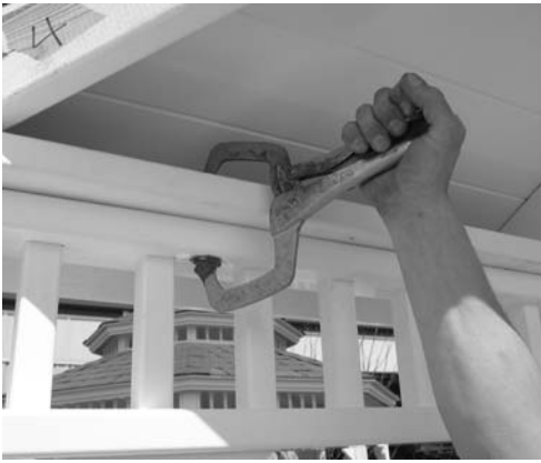
Step 21: Fasten with clamp to temporarily hold roof section in place.
