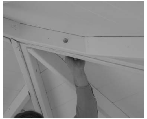
Step 29: Align roof sections and bolt tightly using ratchet set.
