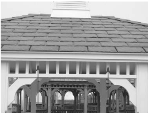
Step 32: Drive 2 (#5) screws on outside of top railing at third spindle from end.
