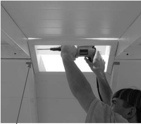
Step 30: Install roof vent from top down (keeping nice side on bottom) and fasten with screws. Note: Vent should be flush with bottom of ridge.
