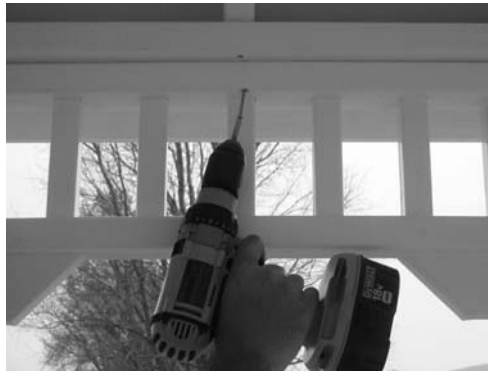
Step 33: Drive 1 (#5) screw on the inside of railing section at center spindle.
