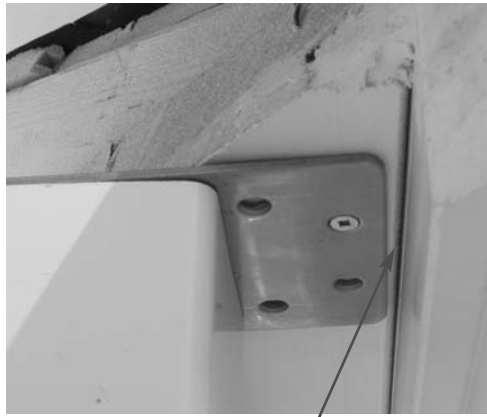
Step 22: Fasten top plate to roof section using #3 screw keeping approx. 1/8" gap between top plate and trim piece. You may need to adjust corners later to fit in the side roof sections.
