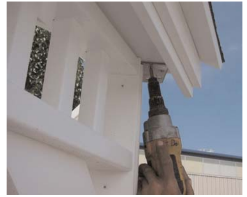
45. Fasten second screw into roof
