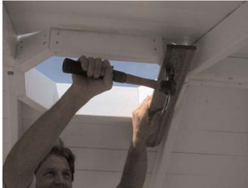
40. Put oval circle into roof hole - you may have to pound with hammer using wood block - never hit finished product with hammer - Make bottom of circle flush with bottom of rafter
