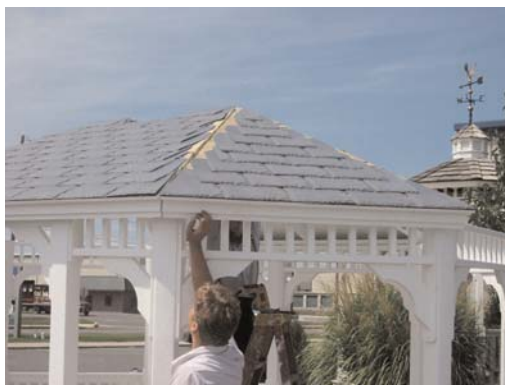
41. Install remaining roof sections matching appropriate numbers
