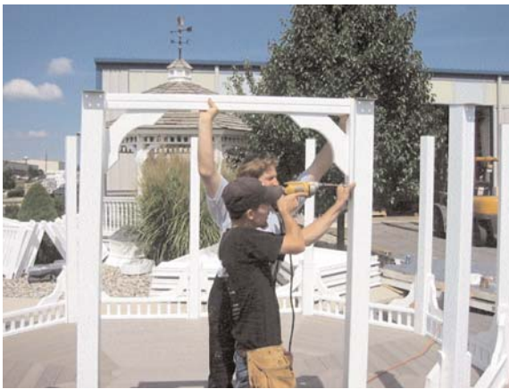
Step 24. This step works well with 2 people - one holding up top railing section while other fastens to post
