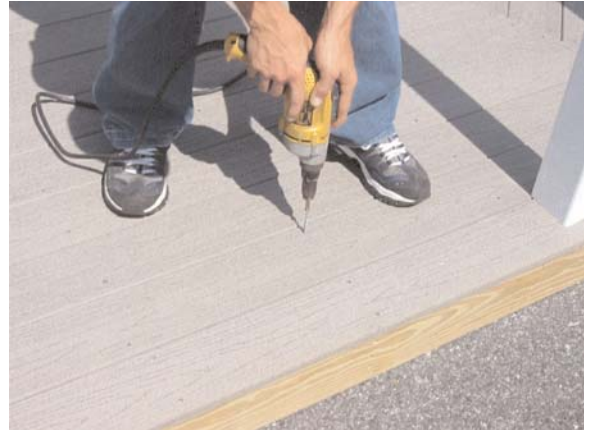
Step 21. Fasten all remaining floor boards with #3 or #4 screws
