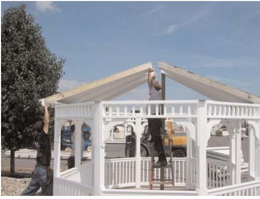
37. Slide 2nd large roof section into place and repeat above steps
