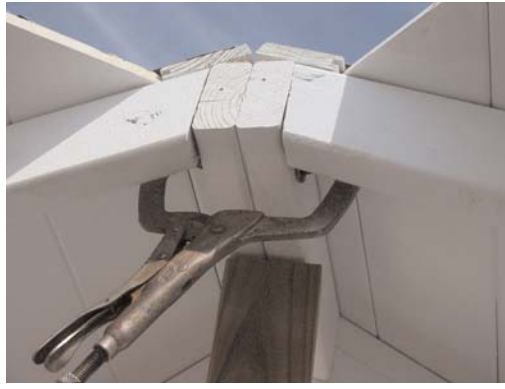
38. Use vise grip clamp to hold roof sections together
