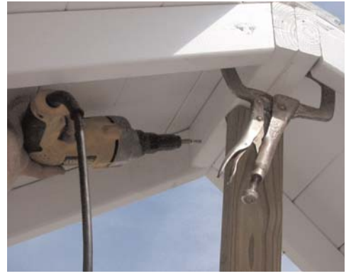
39. Screw rafters together
