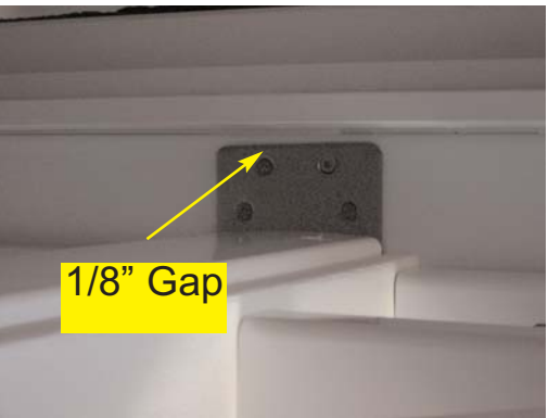
47. Fasten top post plates with #3 screws Note: Correct placement of bracket
