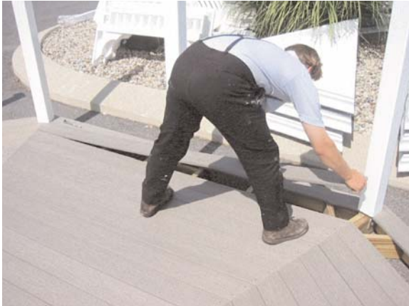
Step 19. Put all floor boards back into place
