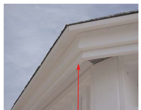
42. Align corner edges flush
