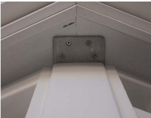
47. Fasten top post plates with #3 screws Note: Correct placement of bracket
