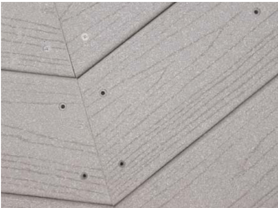
Step 21. Fasten all remaining floor boards with #3 or #4 screws
