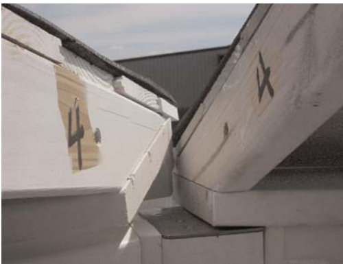
41. Install remaining roof sections matching appropriate numbers
