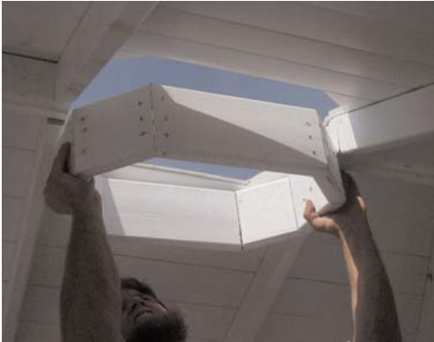
40. Put oval circle into roof hole - you may have to pound with hammer using wood block - never hit finished product with hammer - Make bottom of circle flush with bottom of rafter
