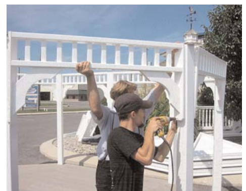
Step 27. Continue with all top railing sections until complete
