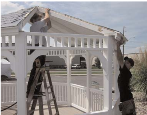
46. Repeat previous steps to install additional roof sections
