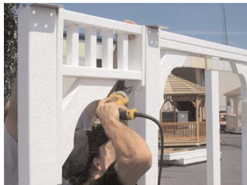
Step 26. Fasten railing section with 4 screws on either end
