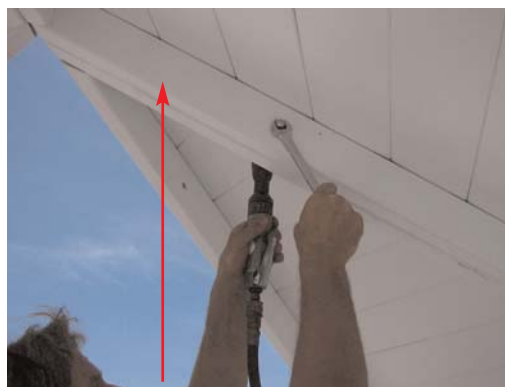
44. Be sure to make rafters flush
