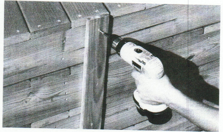
#5 - With floor panels and all other components safely placed where convenient, remove vertical straps holding floor sections in place.
