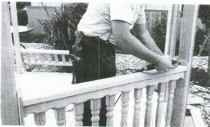
#17 - Install lower railing section with vertical plate resting on deck and centered on post. Note that there are (4) screws in each plate.
