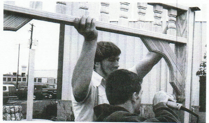
#16 - Position and secure top railing sections in each opening aligning as in previous step.
