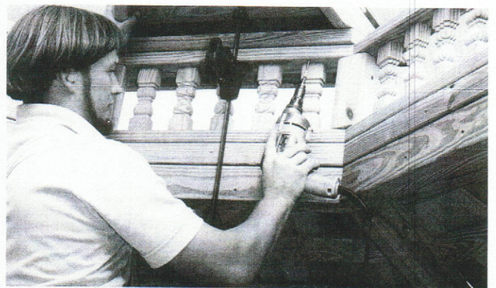
#36 - Screw in place through the railing plate into the roof section.
