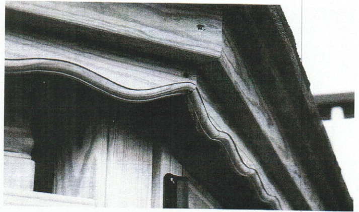
#50 - Adjust the trim corners so that they align as shown and secure.
