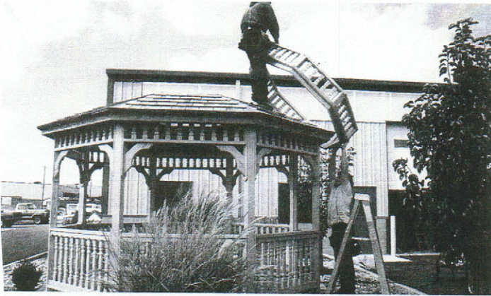
#31 - With assistance, raise the railing section onto the roof and position as shown in hole.
