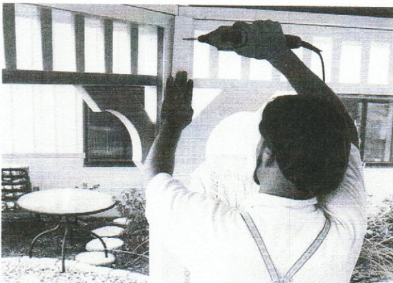
#46 - To install screens, center the panel in the opening opposite the door. Secure the screen panel in place using the "T" shaped trim shown in the next illustration (1).
