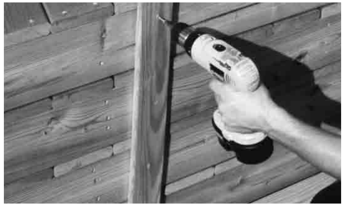
#5 - With floor panels and all other components safely placed where convenient, remove vertical straps holding floor sections in place.
