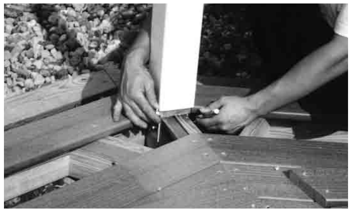
#11 - Insert bolts through post/joint bracket and tighten fully, making sure that outside corners of floor sections are properly aligned. (See #12)
