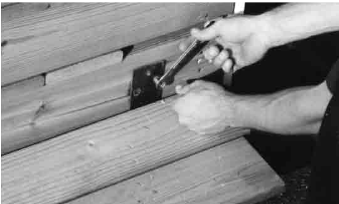
#6 - Remove lag bolts holding floor sections to the skid.
