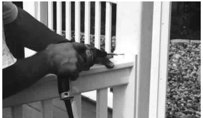
#19 - Install lower railing section with vertical plate resting on deck and centered on post. Note that there are (4) screws in each plate.
