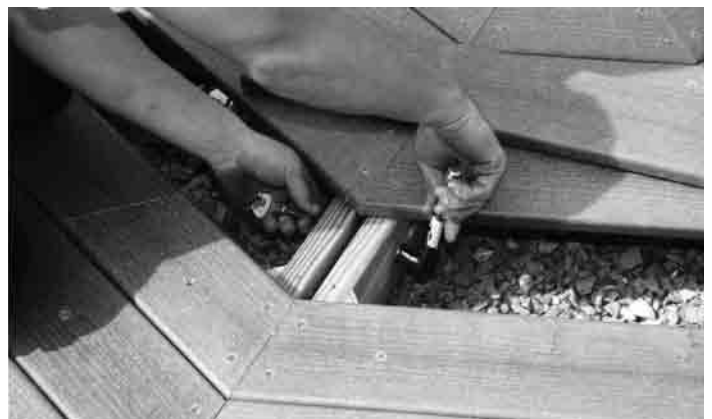
#13 - With post bolts fully tightened insert bolts through pre-drilled holes in joist at floorboard #8 position and tighten fully, making sure that floor boards are flat with each other.
