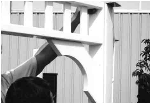
#18 - Position and secure top railing sections in each opening aligning as in previous step.
