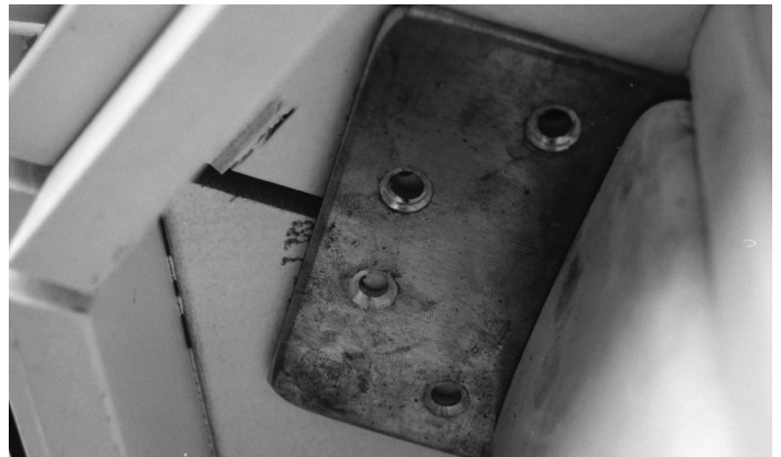
#32 - Do not put screws through roof brackets into 2x8 plate on last corner of panel #7 – next to last panel, until panel #8 is installed and aligned. Panel #8 is placed from the outside of the gazebo.
