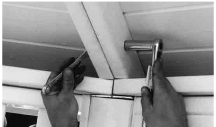
#P9 - Tighten lower bolts first.
