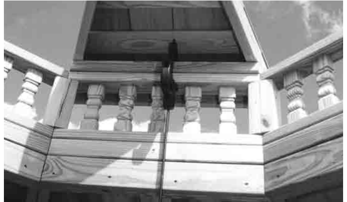
#P5 - With the railing assembly secured, position a roof section and temporarily clamp in place.
