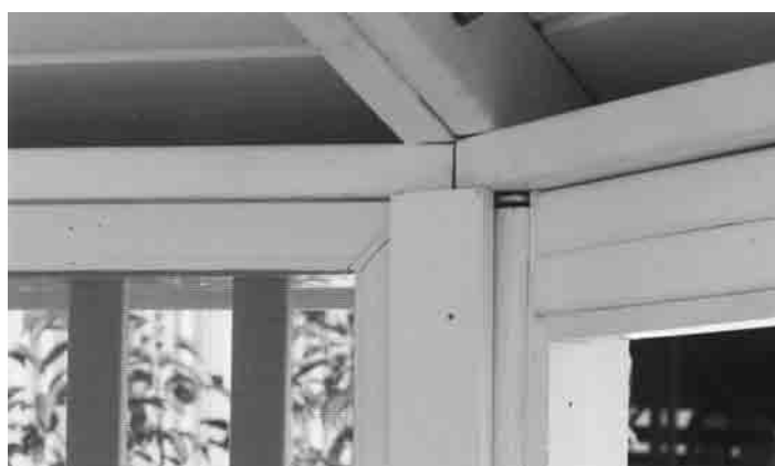
#40 - Finish the screens at the door securing the last panel with trim (2) shown in the previous illustration.
