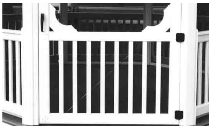
#42 - Adjust the door stretcher so that the door is properly aligned.
