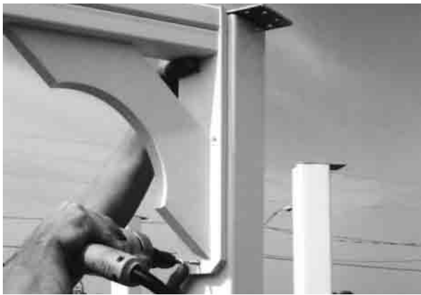
#16 - For gazebo kits without screen package, position header in doorway with top aligned with top of roof bracket and vertical plate centered on post, fasten with screws.
