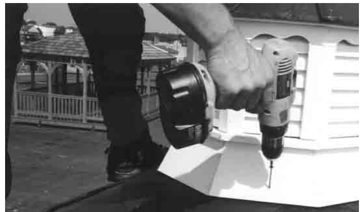
#38 - Align cupola with seams in roof and secure with screws. Check from ground level to insure that the cupola is relatively plumb.
