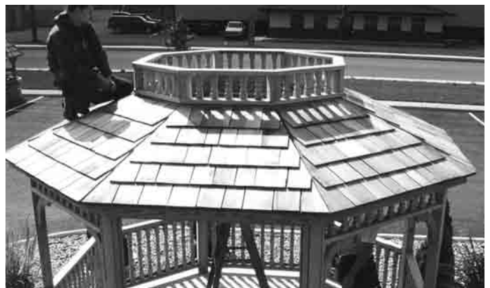
Ready to be secured.
