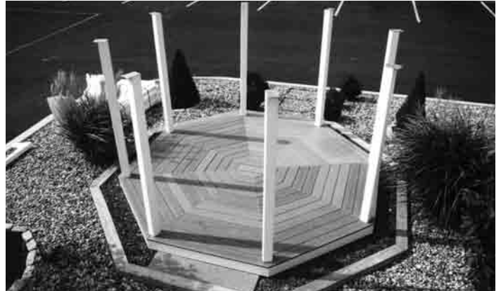
#15 - Deck and posts completed.
