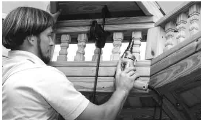
#P7 - Screw in place through the railing plate into the roof section.
