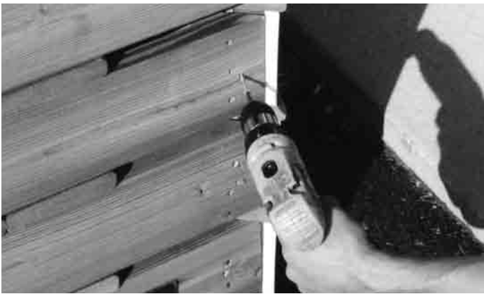
#4 - Each floor section is screwed to another to stabilize the package. Remove those screws.
