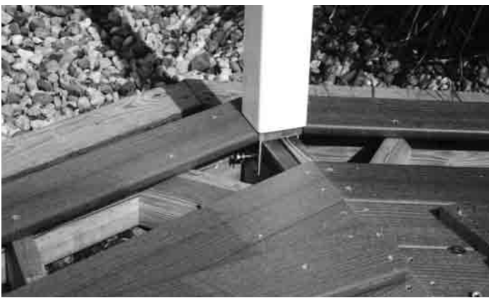
#10 - Place posts making sure that roof brackets are facing out-board (See #15) and post is fully seated on floor joist.
