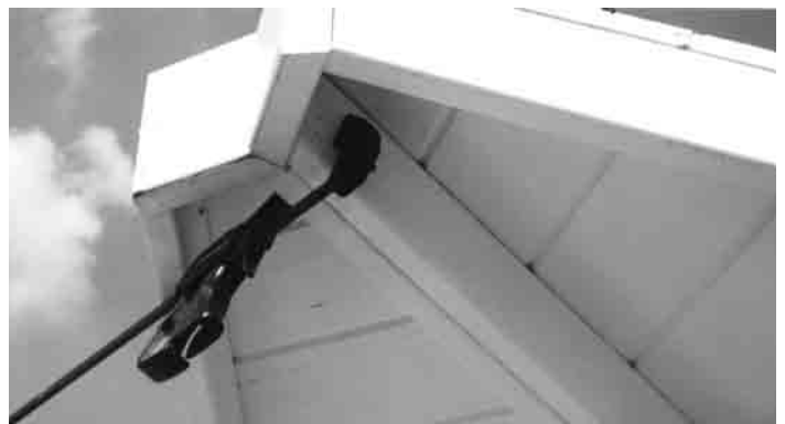
#30 - Align roof rafters with each other and clamp in place.
