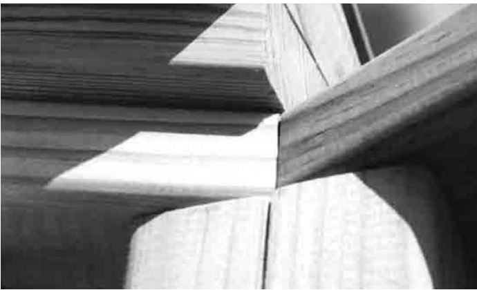
#P6 - Align the panel so that the bottom plate is at the position shown above. Both ends of the roof section plate should be the same distance from the railing plate.
