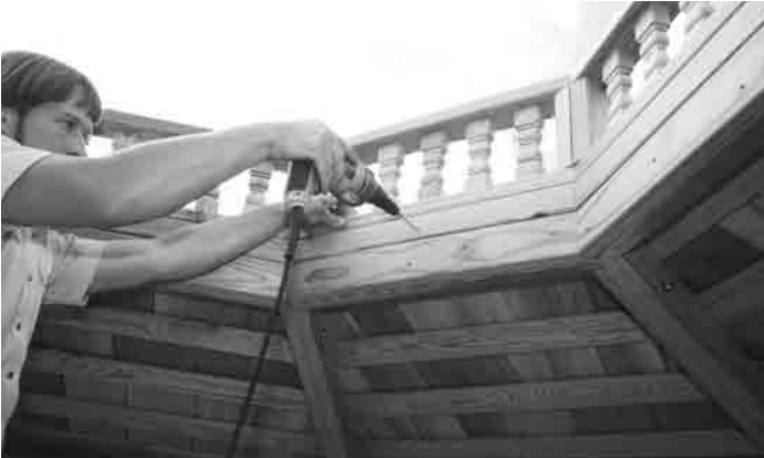
#P4 - Measure from the bottom of the edge of the roof opening to the floor to ensure that each section is an equal distance from the floor. Secure ring in place with screws.
