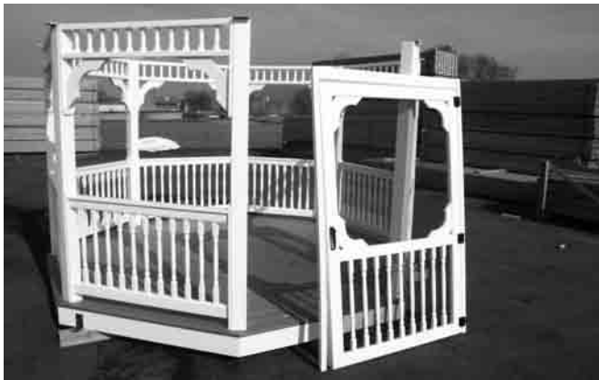
#20 - With bottom and top railing in place and secure, position door assembly in opening.
