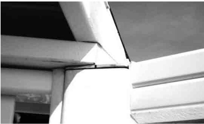
#27 - From inside of gazebo place roof section so that the corner of the 2x8 roof plate is on the center mark of the post roof bracket.
