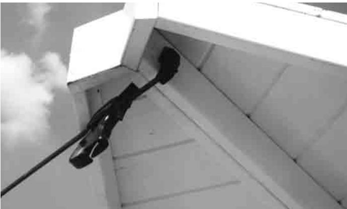
#P8 - Position next section aligning rafters and bolt together.
