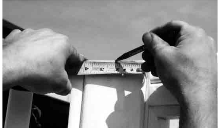
#26 - Determine center of roof bracket and mark.
