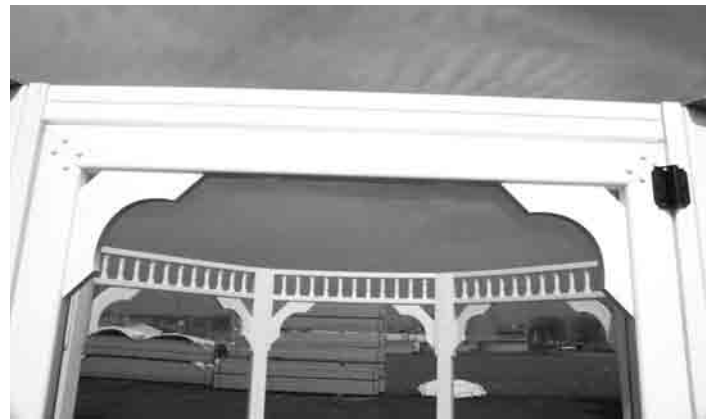
#23 - Properly installed the door top edge and side edge are parallel to the jamb.
