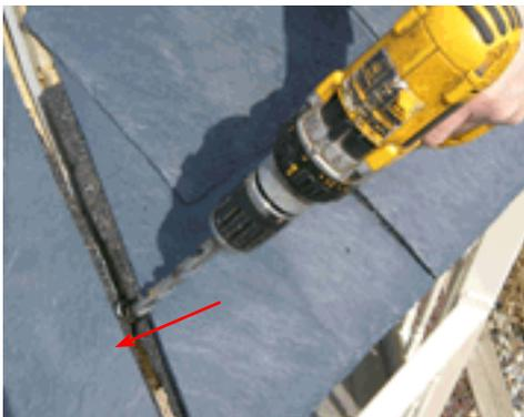
Step 3: Pre-drill wire hole from top of roof down through rafter on hard angle.
