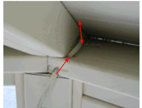
Step 2: Pre-drill wire hole at top plate as shown.
