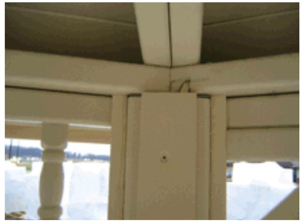
Step 5: Install wire trim strip with 4 screws into pre-drilled holes.
