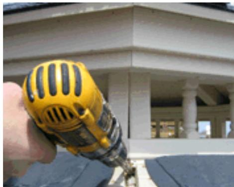
Step 4: If you have purchased a double roof gazebo, pre-drill wire hole starting directly on top of rafter and through top 2x6 ring.
