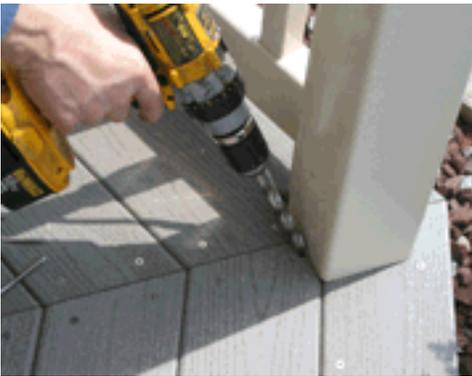
Step 1: Pre-drill wire hole using 5/8" drill bit. Start drilling 1/2" away from floor splice towards door way, **angling at a hard angle towards door way through 4x4 post below floor surface (this is very important).**
