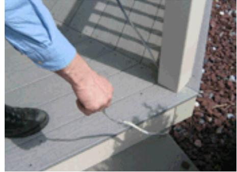
Note: After bottom steps are completed there should be at least 18" of wiring from bottom of floor.
