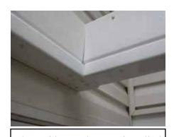
Place Side Header onto installed Header Plate (as shown). Install Posts on opposite end as shown in Pergola assembly manual.
