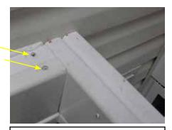
Fasten Top of Headers together using (2) 2.1/2" Panhead screw, toed (Shown with yellow arrows). Install opposite side header by repeating previous 3 steps.
