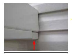
Ensure Header is Flush at bottom and fasten using (4) 2.1/2" Panhead Screws (as shown with red arrows).
