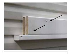
Attach 2nd 2x6 Board to the Header Assembly to cover screws going into house wall (as shown). Using 2.1/2" Pan Head Screws every 16" threw pre drilled holes alternating one near top and one near bottom.
