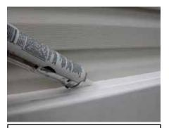
Apply Caulk at top of header and house wall to prevent water from running behind Header Plate. And also to keep water from entering house wall through screw holes.
