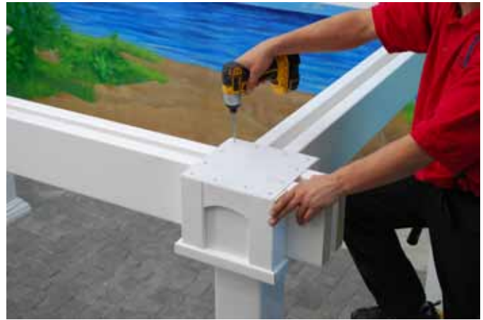
Fasten to pieces below using (12) 1" Pan Screws. Adjust trim pieces to fit snug against header when fastening.
