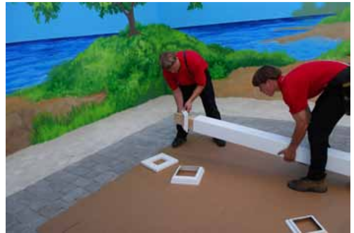
Insert all Trim Pieces onto post from the top of the post down.
