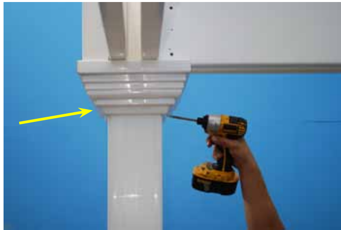
Fasten to post on 2 opposite sides with 1 screw per side.
