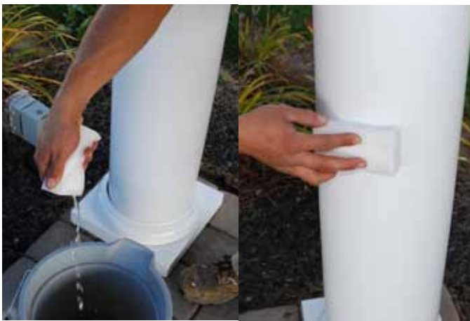
Using the provided Mr. Clean Sponge, dampen with water and use on all vinyl areas to clean any scuffs or dirt that may have happened during installation.
