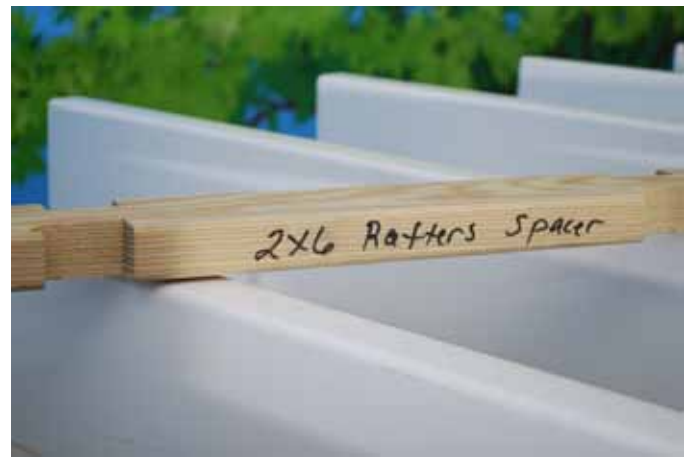
Locate Rafter Spacing Board and use the side with 2x6 Rafter Spacer written on.
