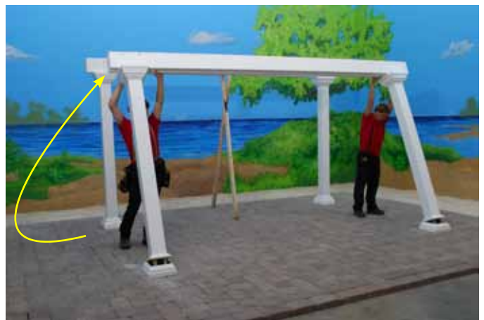
Carefully lay the post side down and lift the header side up into an upright position with the Nibs on the Main Header facing the inside of the pergola.
