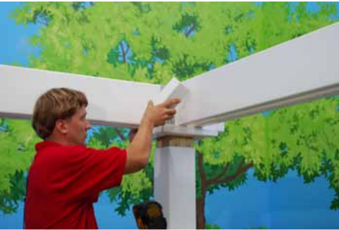
Install Inside Corner Trim.
