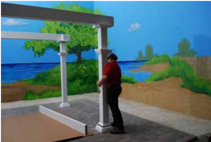
Adjust Posts to appropriate distance apart.
