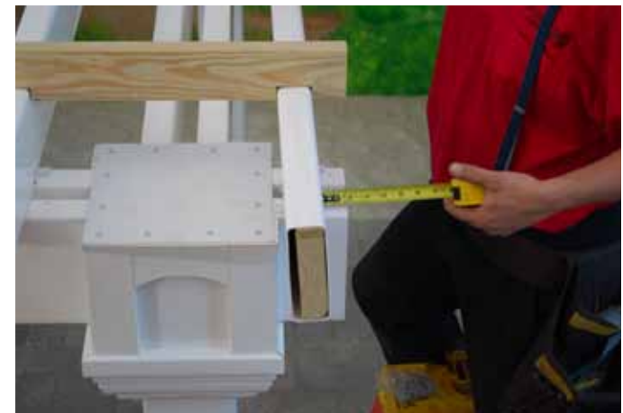
Measure both ends to create equal spacing.
