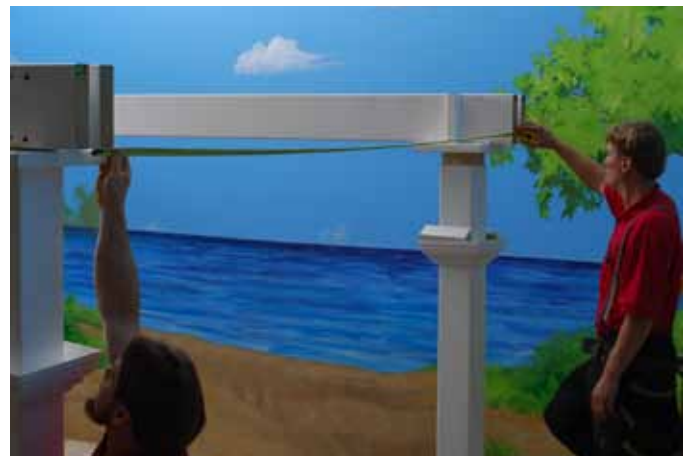
Measure spacing distance between the two Header Assemblies.
