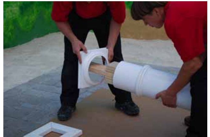
Insert all Trim Pieces onto post from the top of the post down.
