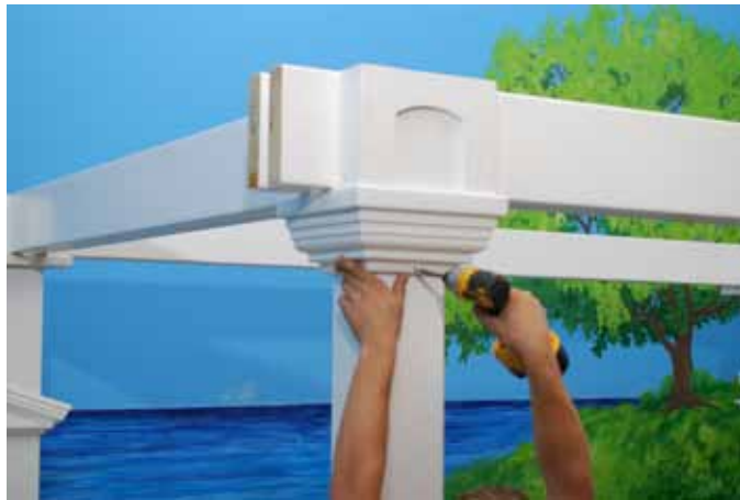
Fasten into post using 2" Pan Screws.
