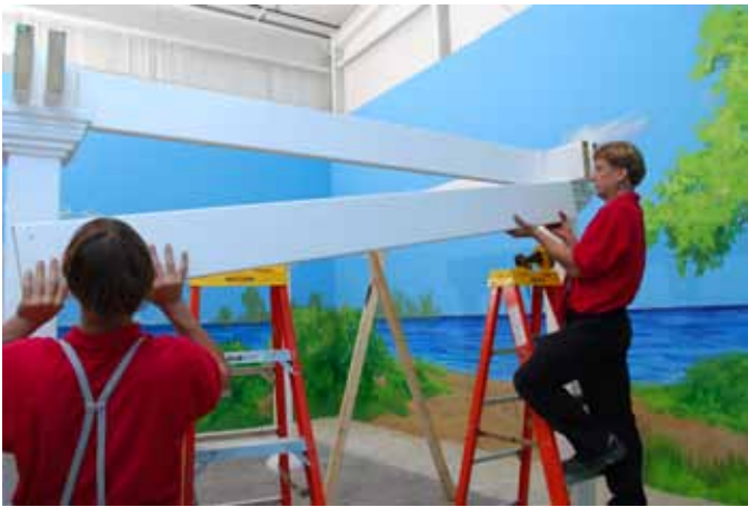
Install 2x8 Header on outside.
