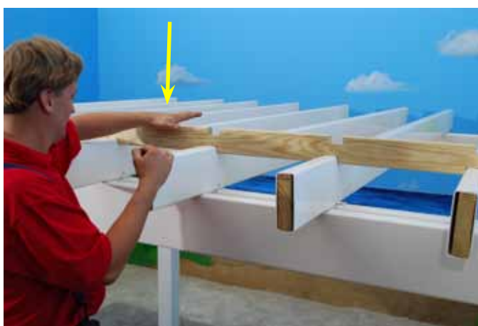
Tap spacer firmly down into place.
