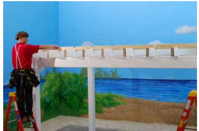
Starting at one end, slide each Rafter into position at each notch in spacer.
