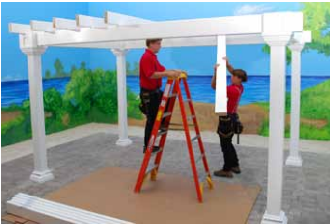
Set all 2x6 Rafter Joists into place.
