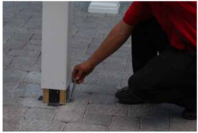
Insert provided 4" Concrete Lag or purchase longer ones if your piers are below pavers. Be sure to have a bolt long enough so that at least 4" of the bolt is firmly into concrete footer.
