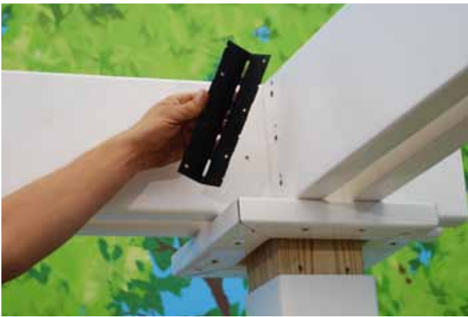
Install Corner Brackets on the inside corner
