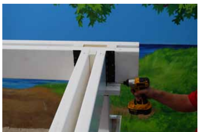
Install Corner bracket on outside corner
