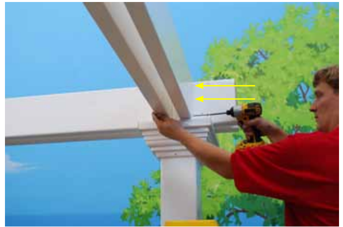
Fasten using (3) 3.1/2" Brown Screws.
