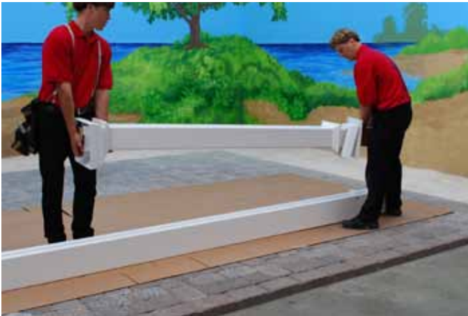
Install Post with trim pieces already in proper place. Note: All Trim Pieces must be installed on the post before completing this step.
