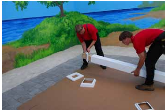
Insert all Trim Pieces onto post from the top of the post down.
