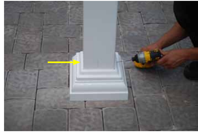
Slide both Trim Pieces down against ground. Push Small Bottom Trim down to pop onto lower Large Bottom Trim Piece. Attach to post using (2) 2" Pan Screws. One on both sides opposite each other.
