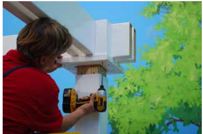
Fasten Square Trim to outside Corner Trim from the bottom up using (1) 2.1/2" Brown Screw.
