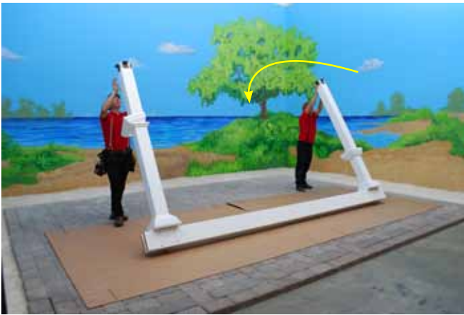
Lower Posts of the header assembly.
