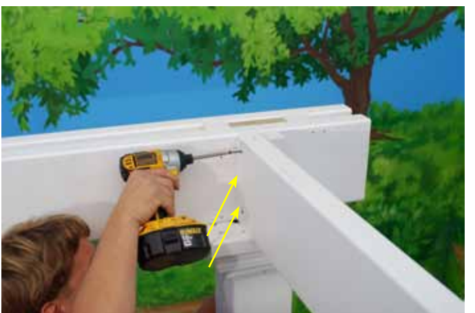
Attach 2x8 header to Nibs on Main Header using (3) 3.1/2" Brown Screws.
