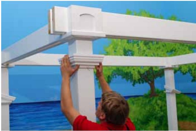
Slide both Top Post Trim Pieces tight up against Square Trim Piece.
