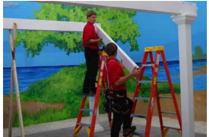
Install 2x8 Header on inside.
