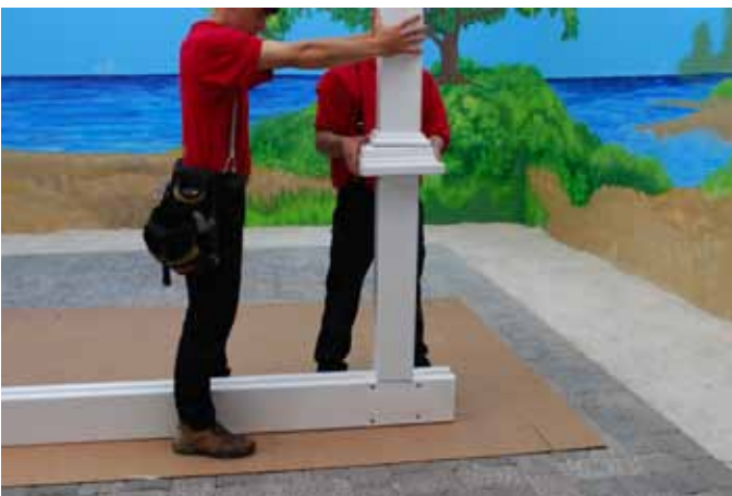
Slide post down against and hold in a level position.
