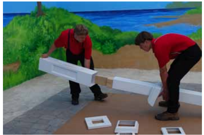
Insert all Trim Pieces onto post from the top of the post down.
