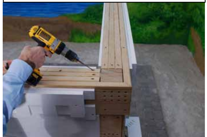
After all headers are up and installed, fasten top side of Top Header to Post using 3.1/2" Brown Screws (toed).
