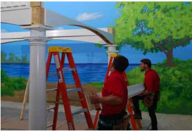
Install the shorter Top Header
