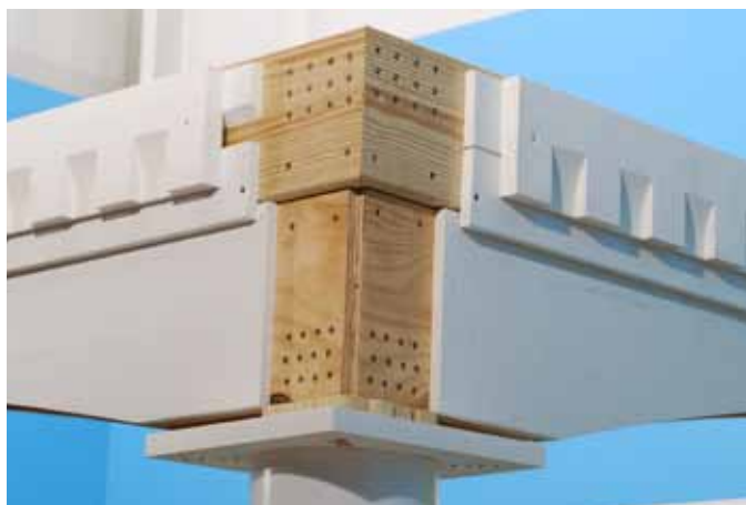
Fill Pre-Drilled Holes along edge that were left empty in previous steps. This is where you should be now. Install opposite side using the prior steps.
