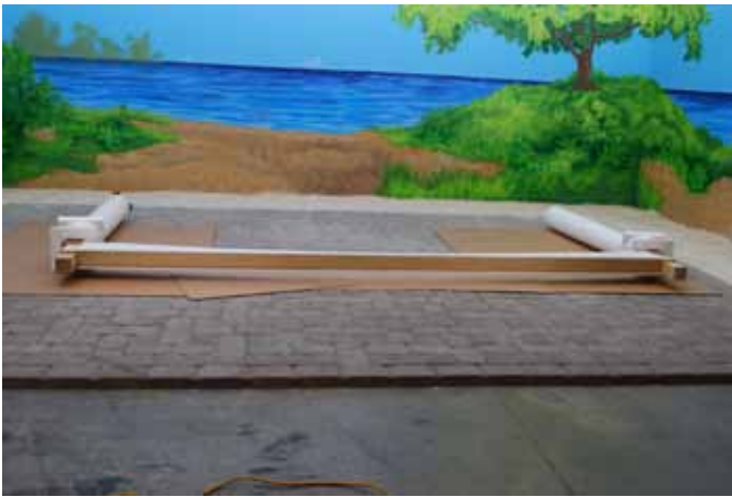
Photo of first Arched Header attached to both posts.
