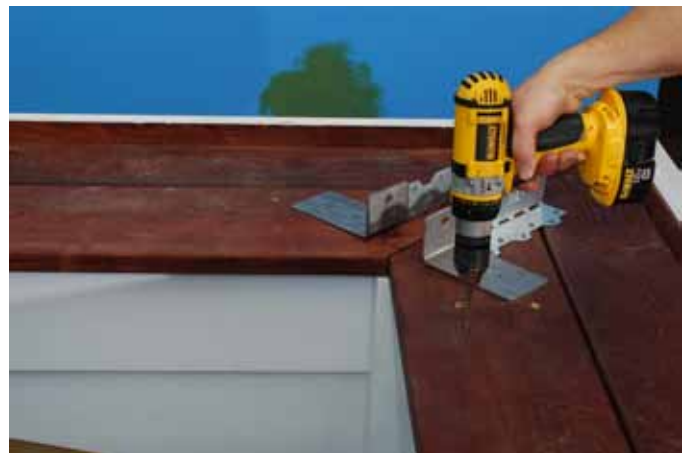
Fasten Roof Plate temporarily using (1) 3.1/2" Brown Screw at each end in the location shown. This is NOT pre-drilled.
