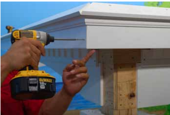
Fasten corners together using (1) 2" White Head Screw per corner. This is not predrilled.
