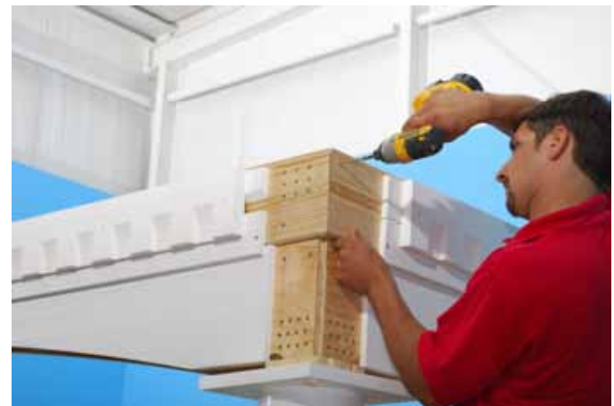
Fasten Top Header using 3.1/2" Brown Screws into every pre drilled hole.
