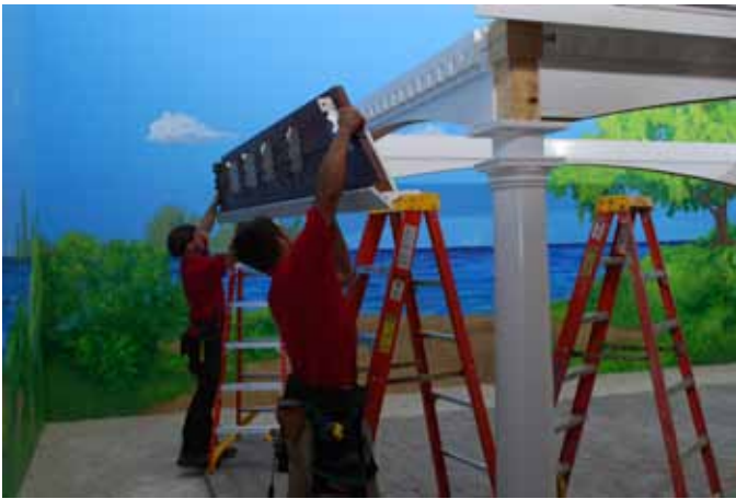
Install adjacent Roof Plate.
