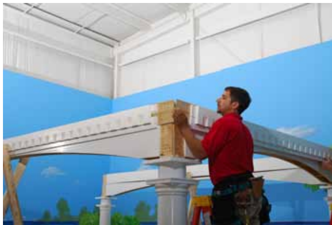
Place Top Header on top of Arched Header and align evenly at corners. Ensure snug fit against post and Arched Header.
