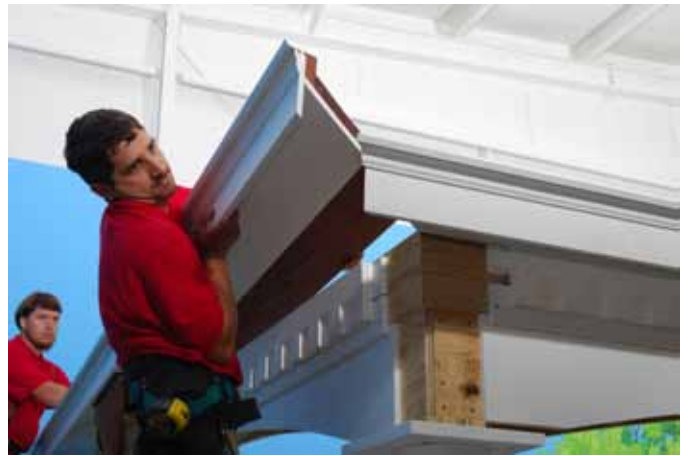
Place Roof Plate into position
