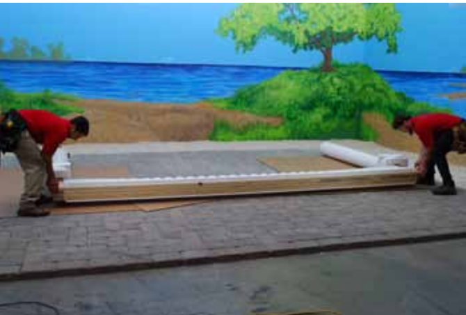
Place Top Header into position with dental molding faced up. Top Header should slide into position snug against Arched Header.
