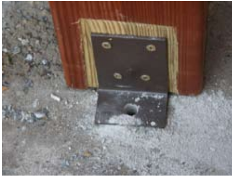
Photo Showing Newly Drilled Hole.
